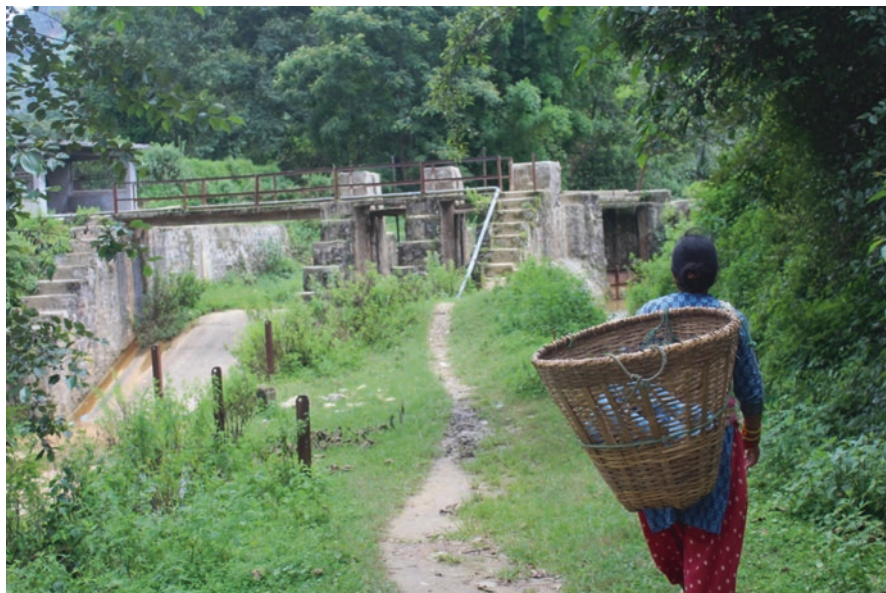
Fig. 3.2 Dam of Mahadev Khola Rajkulo. (Photo Anushiya Shrestha)
